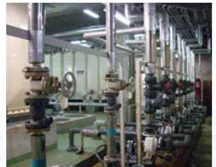
Natural seawater (taken from the port of Ooigawa and filtered) and groundwater (drawn from 120m depth) are supplied continuously to the laboratories of the institute.
