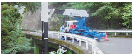
Inspection/diagnosis by bridge inspection vehicles
